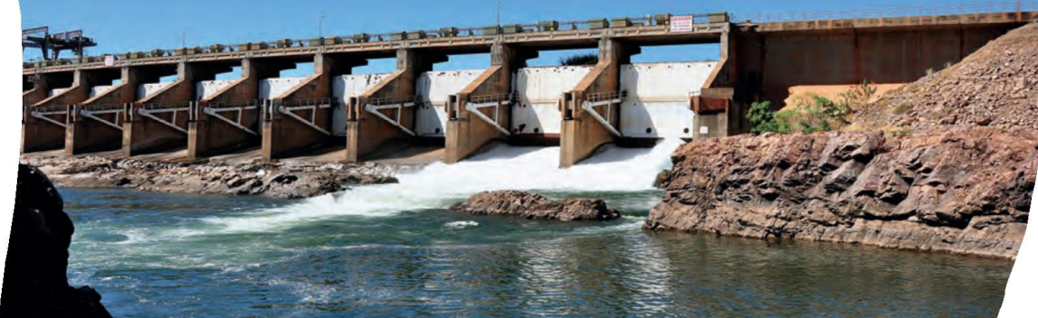
Water discharging below the Diversion Dam on the Ord river, Kununurra, WA Credit – Angus MacGregor and the Department of the Environment
